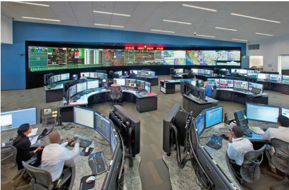
Figure 4-2. Contemporary control room circa 2014 illustrating the human-machine interface (HMI) configurations for each individual operator as well as the large shared displays for coordination and overview.
