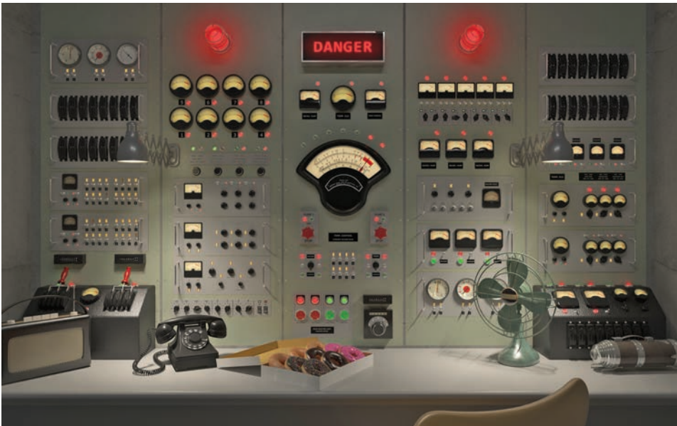
Figure 4-1. Early control room, circa 1950 design. Note the presence of important indicators yet few controller stations. The operator was expected to be able to gain a good overview of the entire process by “eyeing the board.”
