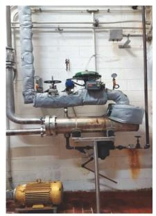
Figure 3. A Midwestern cheese manufacturing plant "before," using an automated ball valve and a range of improper practices. Source: KEI Steam Solutions, Inc.
