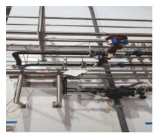
Figure 4. The cheese manufacturing plant after implementing a rotary control valve and other best practices. Source: KEI Steam Solutions, Inc.
