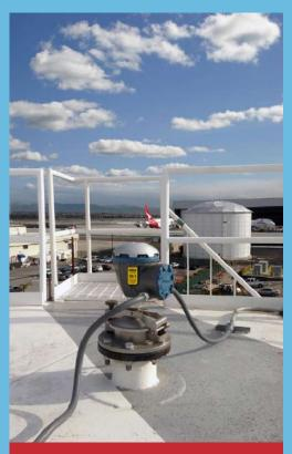
Radar level instruments can be used in hazardous applications such as fuel vessels. (Shown is Emerson's Rosemount 5900S Radar Level Gauge.)
