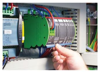
Figure 3. ECPs available in an expandable form factor with convenient bussing make it easier to design and fabricate control panels with many Class 2 circuits.
